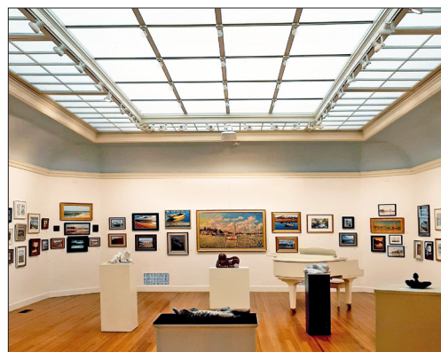
A view of the attic of the Lyme Art Association, with skylights above and laylights below that bathe the galleries in natural light.
